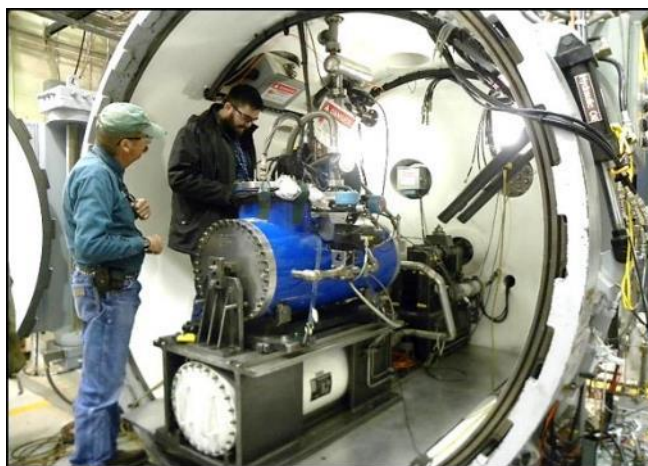
Secondary and Primary Containment Chamber
